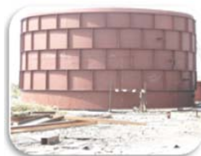
Bunker Shell Fabrication
