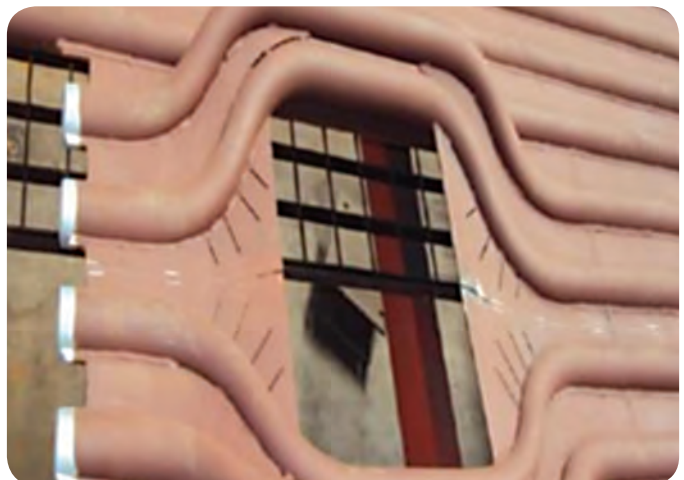
Water wall panel
