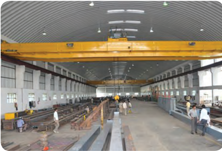
Inner side of the K-55 plant shed
