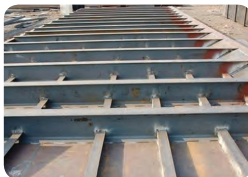
Fabrication of Duct 500 MW
