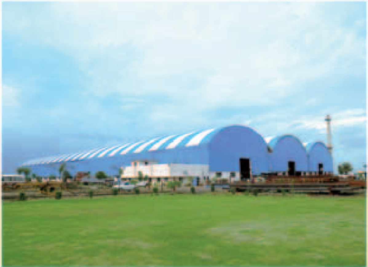
Seam Industries Limited, K-55, Unit-II, Heavy Fab Shop
